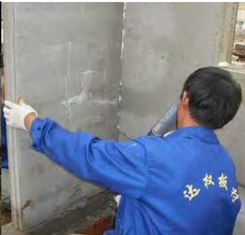
SEAL USING FOAM
